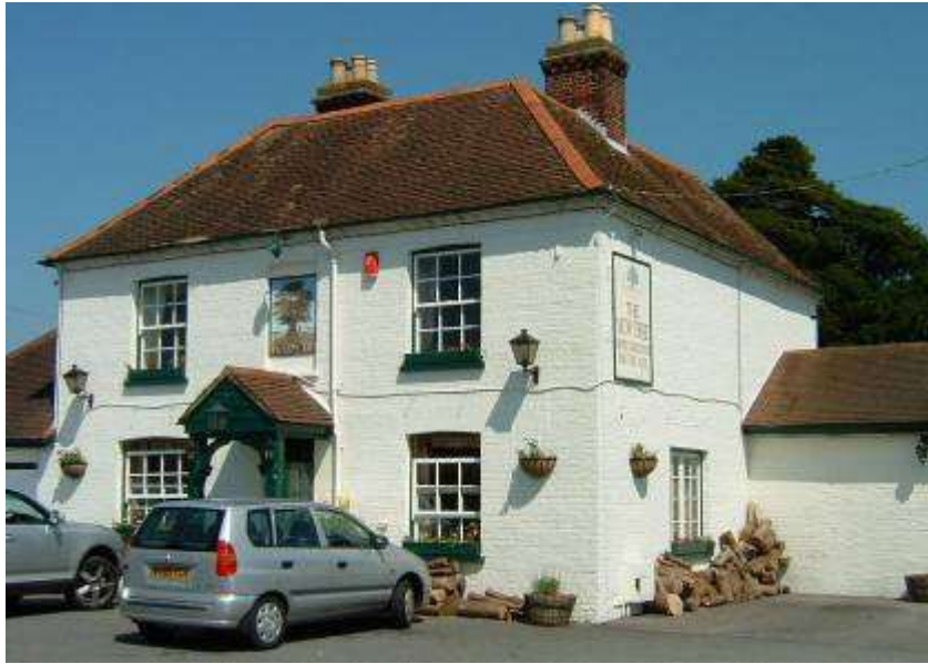
Yew Tree Inn, Hayling Island. Note the tree's canopy at the rear.
